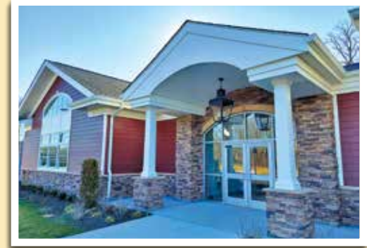
Construction of the new Moriches satellite branch is complete. Books, supplies, and furniture have been moved in. The town has issued its Certificate of Occupancy. We are awaiting final land division approval from the school district.
