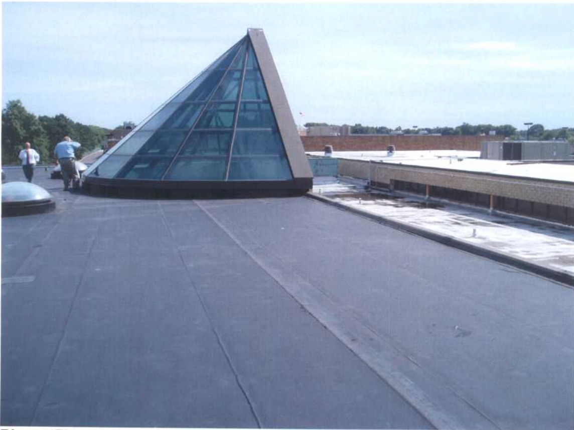
Photo 'F' 1995 –Addition roof skylight
