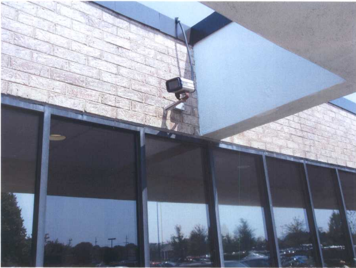
Photo 'C' Typical exterior windows.
