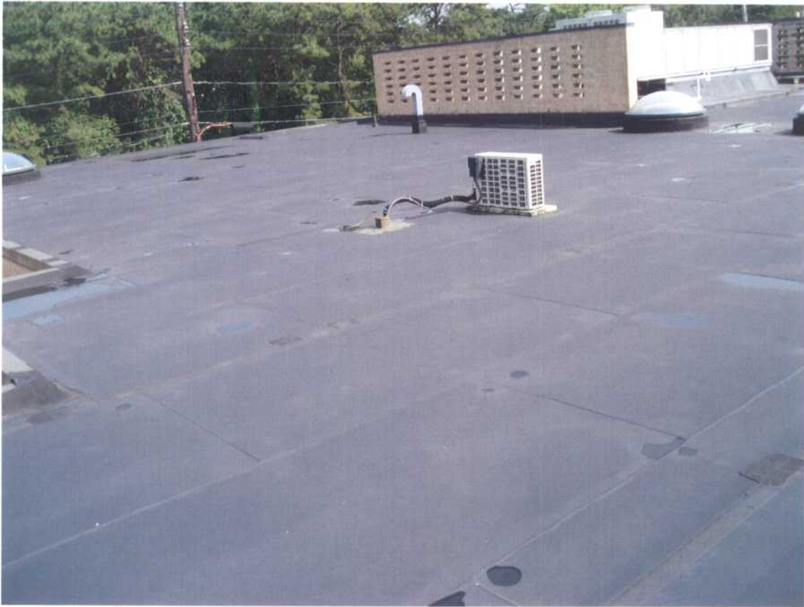
Photo 'E' 1995 –Roof area
