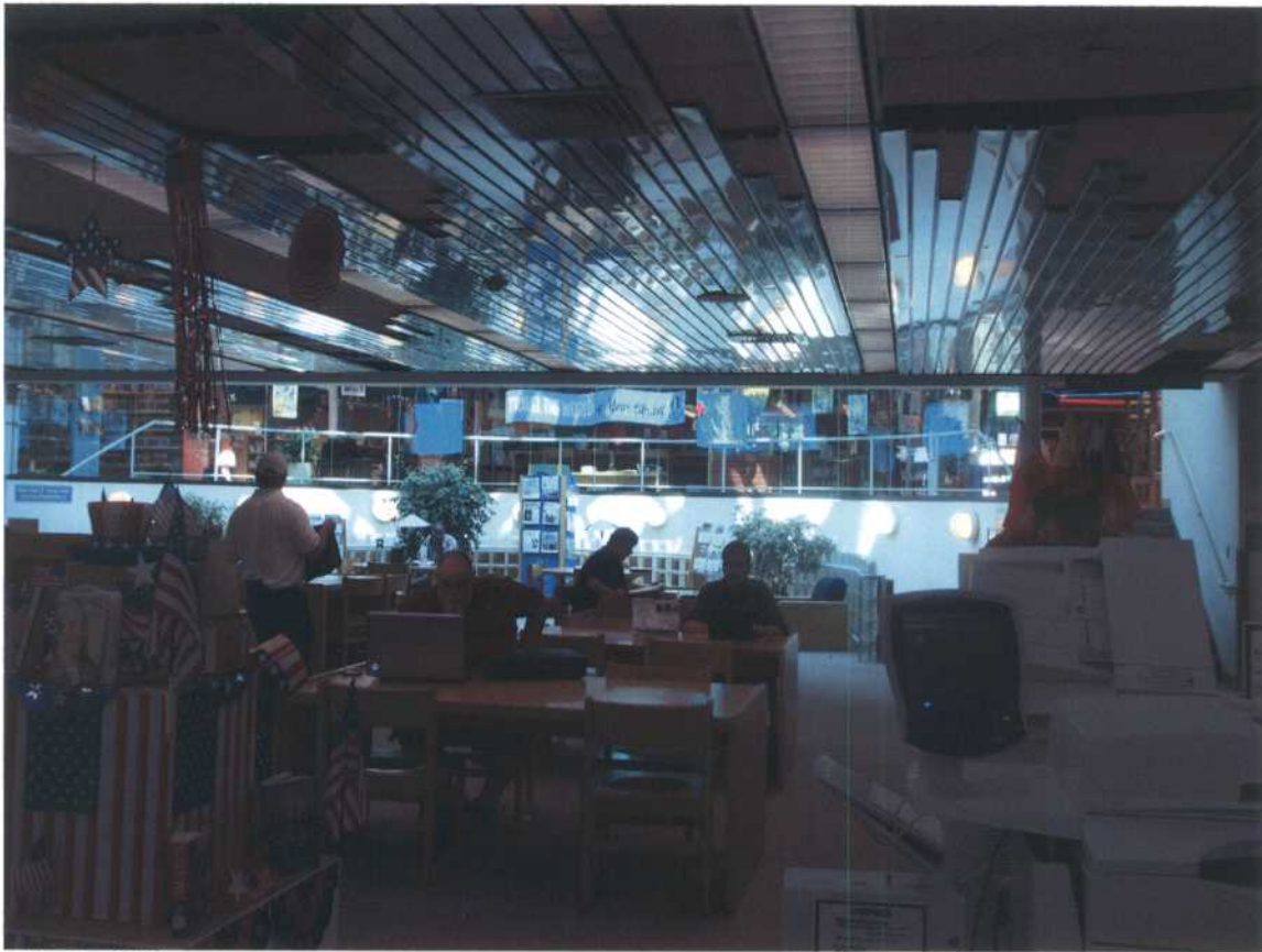
Photo 'G' Existing chrome panel suspended ceiling.
